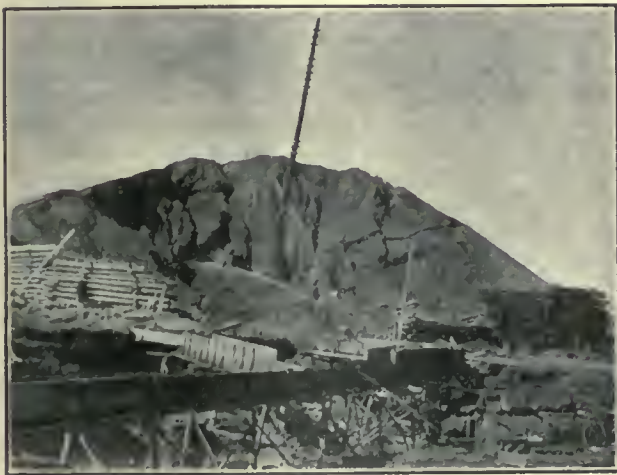
SLUICING A WINTER DUMP, FAIRBANKS.
